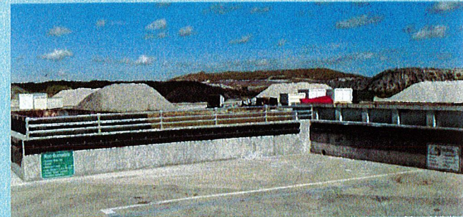
CCDC non-burnable and burnable material bunkers
